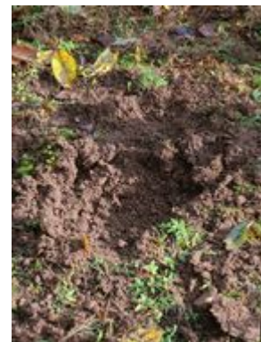
8. Back fill hole left for safety!
