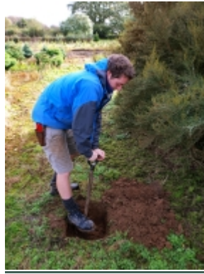
10. Dig and prepare new hole for plant.
